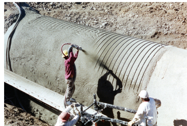
IMAGES: Large diameter water pipelines inspection (top), analysis (middle), and repair (bottom)
